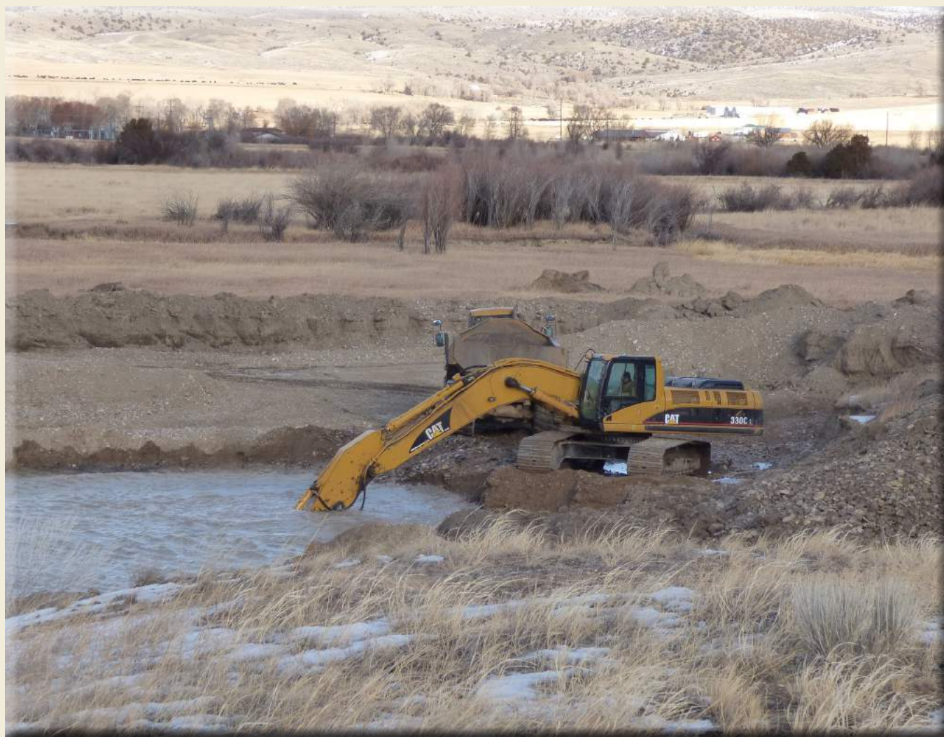
An excavator digs up gravel to place in the streambed. That hole, which will be filled in upon completion, is some 12' deep!
