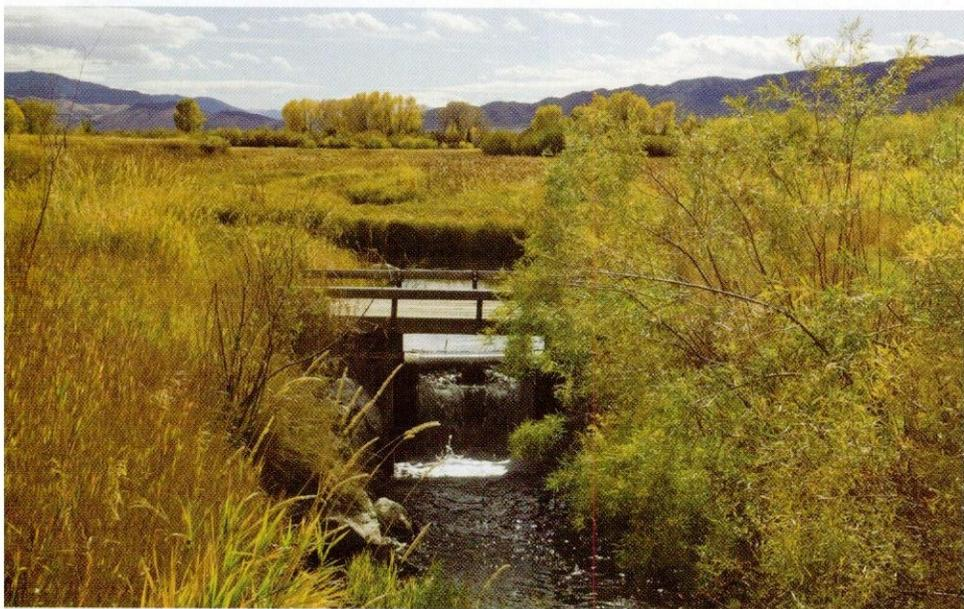
A rolling cylinder aerates water converging from the managed wetland into Clear Creek, a braid of the Ruby River.
